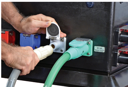
Align the inline Neutral connector with the corresponding color-coded receptacle
