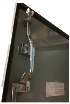
Ensure that the Kirk Key lock properly engages with the catch when the unit is closed.
